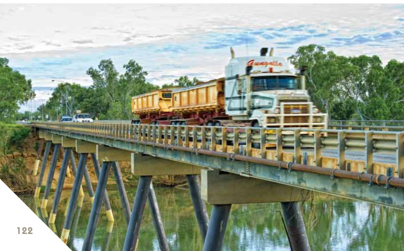
Fitzroy Crossing Bridge.
